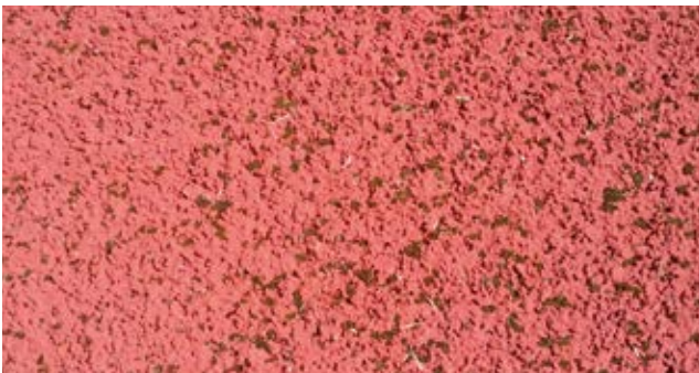
Bad example: Moss-covered synthetic surface
